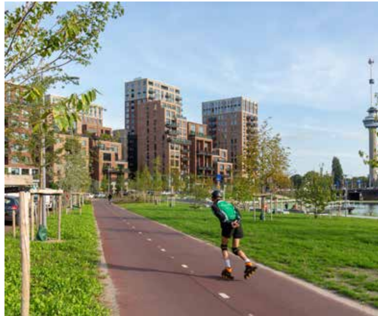
INBO's Little C is part of a major upgrade of the Rotterdam Coolhaven waterfront
