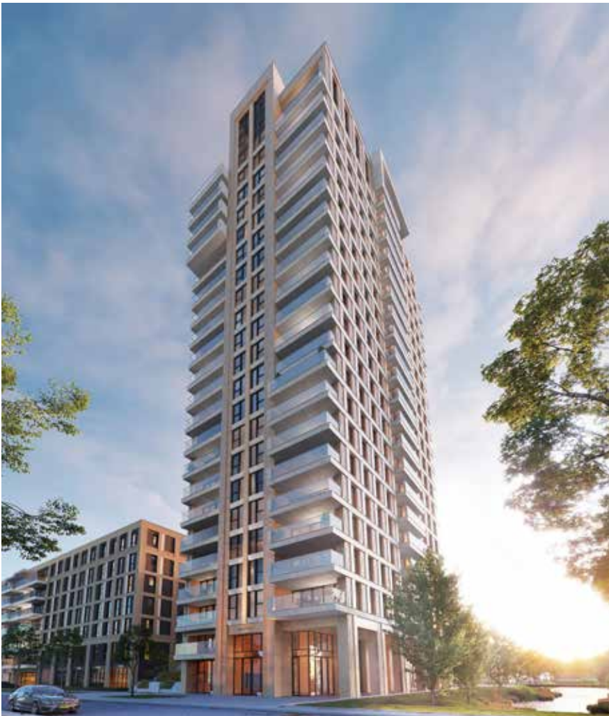
The Maestro development in The Hague is a green building located close to the dunes and beach
